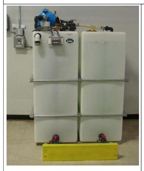
System shown is at Kooltronic Inc. in New Jersey. Their paint line and required emergency shower are on the other side of the wall. By installing this system they avoided upsizing several hundred feet of overhead piping and installing a heater to bring the water to the required 60 degrees F. Plant engineer supplied bumper guard shown.
