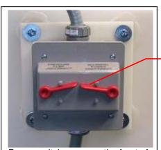
Power switches are on the front of the unit. One switch for the pump and one for the solenoid(s)
